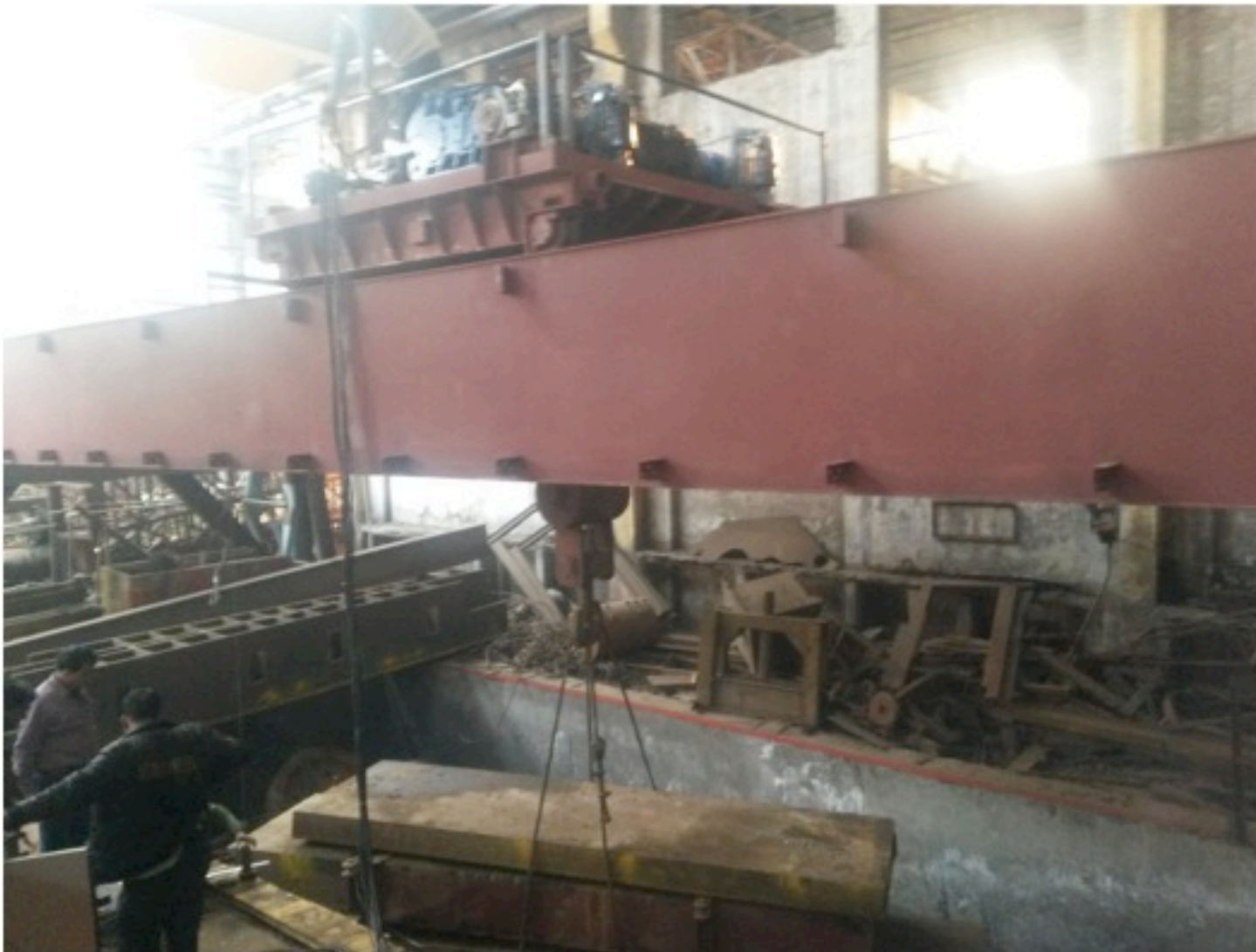
Testing Pit 25 T NTPC Crane under test
